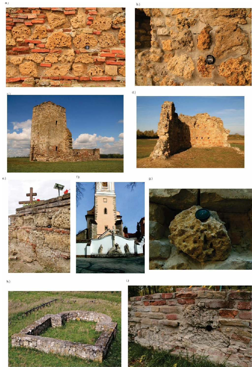
Fig. 1.: Medieval church walls and church foundations built of freshwater limestone of the Danube-Tisza Interfluve, Hungary
