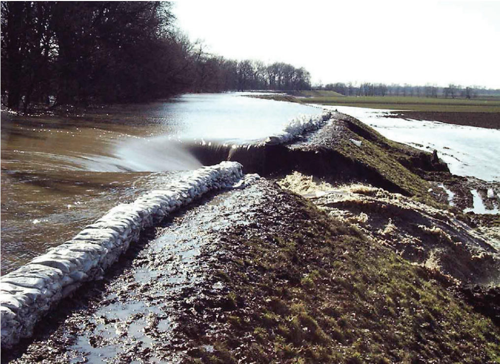
PICTURE 1 ♦ Dam break in Tarpa. (Photo: www.tarpa.eu )
