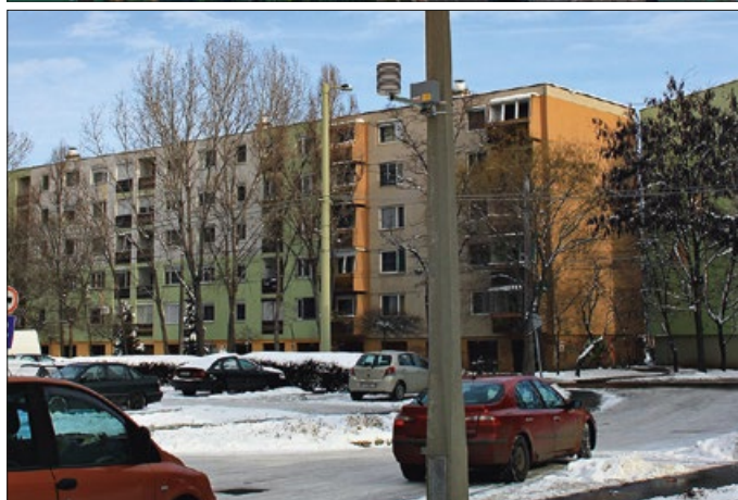
■ Figure 33. Open midrise station location in Szeged
