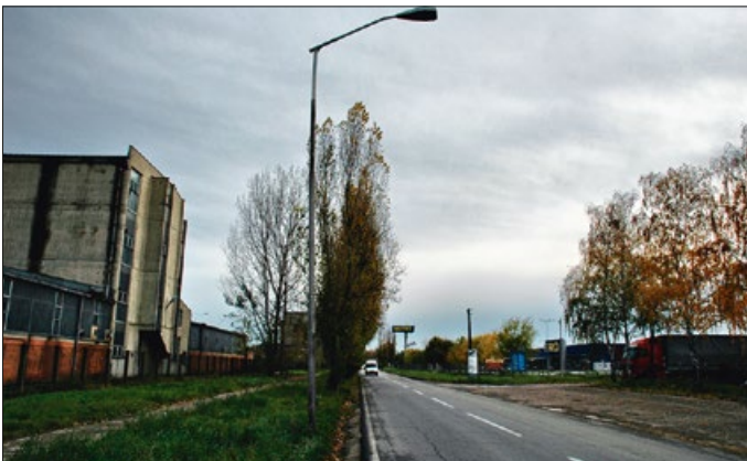
■ Figure 52. Large low-rise (LCZ 8) monitoring station location in Novi Sad (Industrial area –south)
