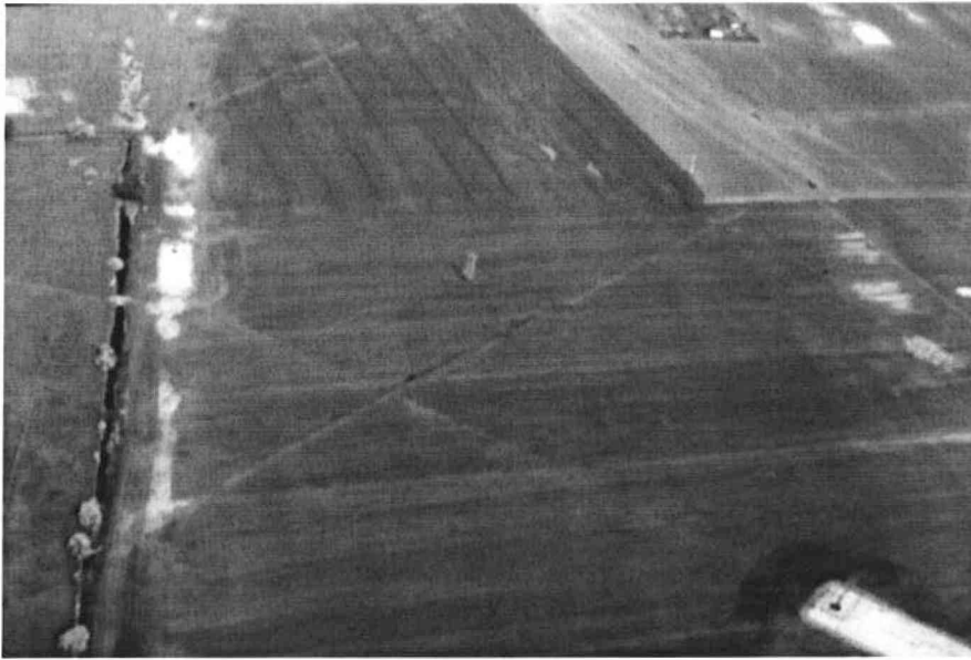
Figure 5 Aerial photography of underground pipelines on the oilfield. On the bottom right corner basement of an oil well can be seen.
