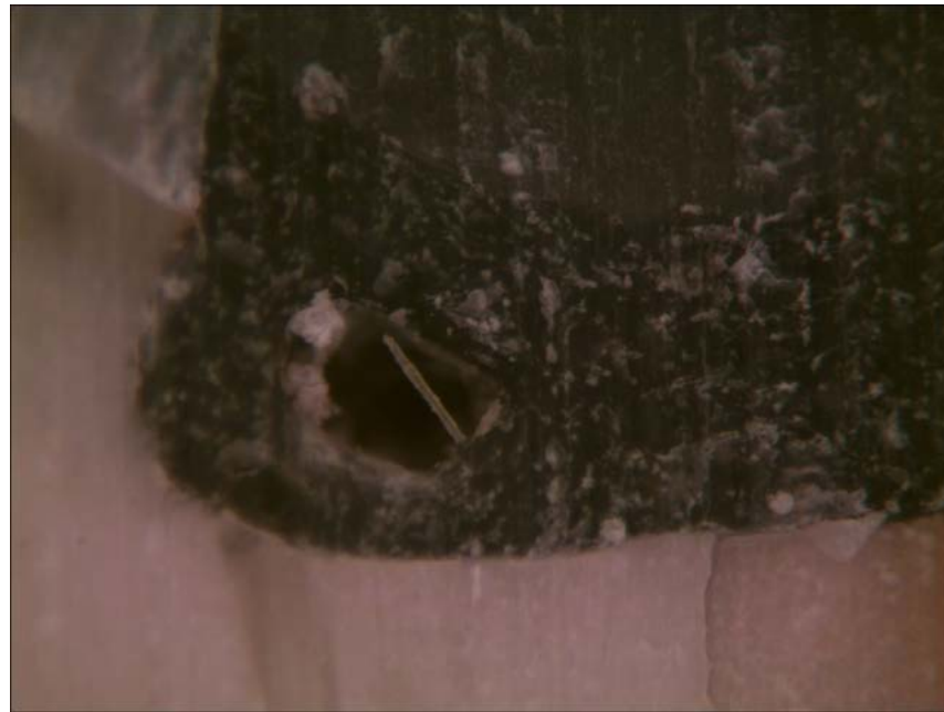
Figure 5. Internal air-bubble formation within the cured SFRC material.
