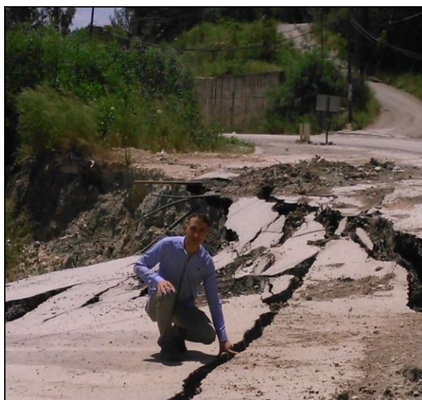
Figure 9. Ground picture of the latest landslide in the study area near to the dam location (March, 2019)
