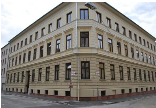
Picture 2.1 Typical tenement building in Budapest from the late 19th century. Source: Zoltán Kovács
