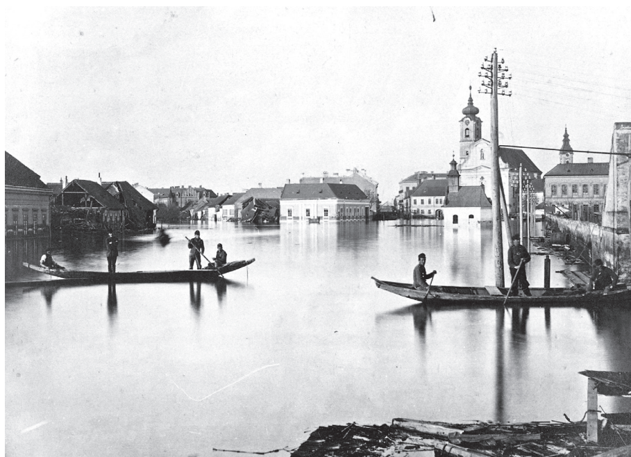
Palánk under water, 1879 (The Votive Church was built on this site in 1930)
